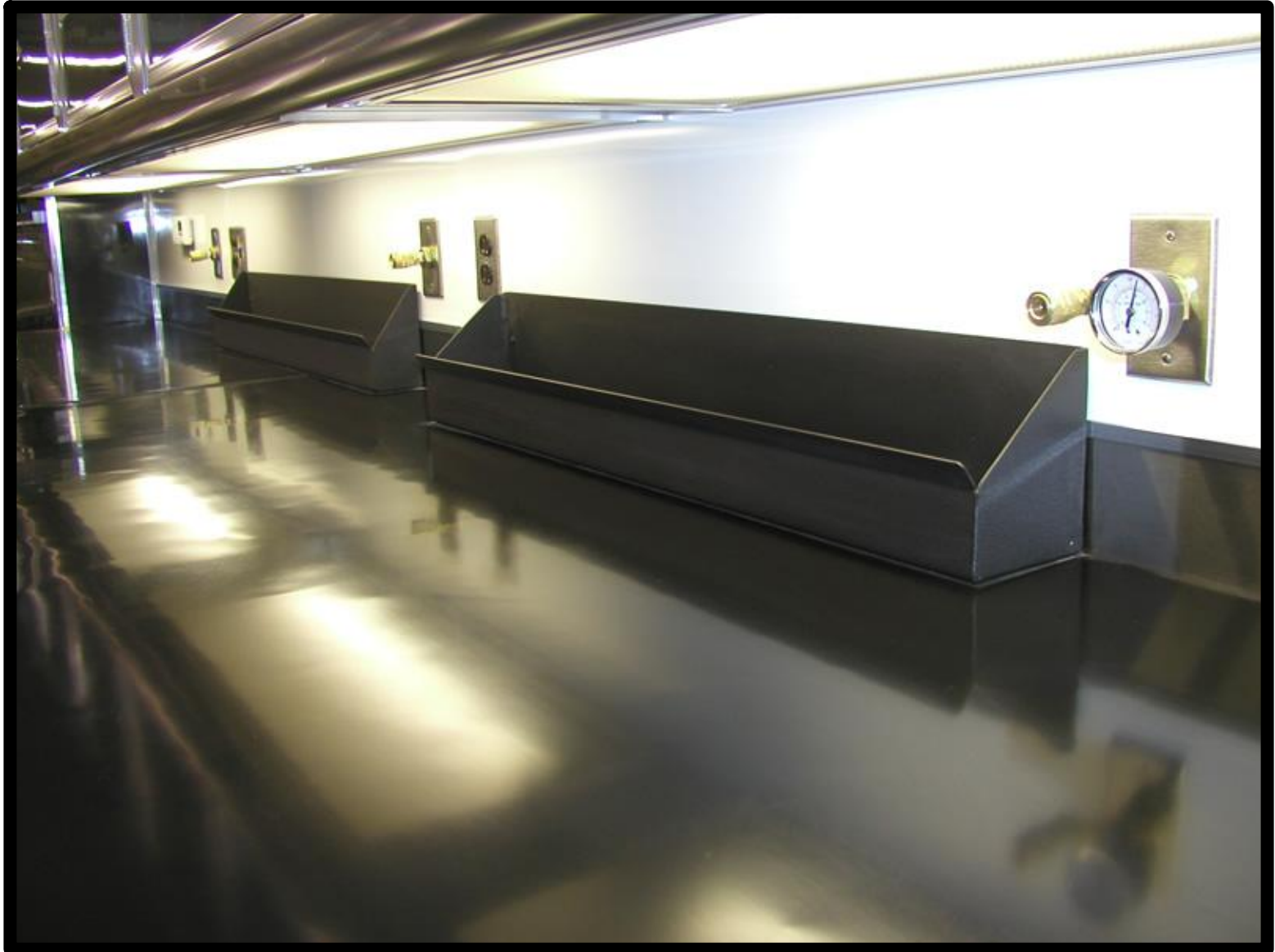
View of main work bench in lower level work area –can racks, rubber bench top
