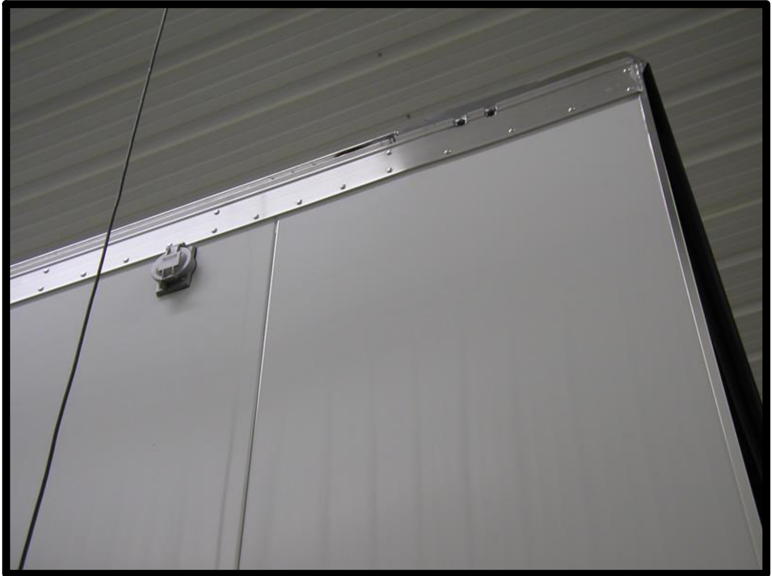
Weather station plug in at top of the rear road side wall
