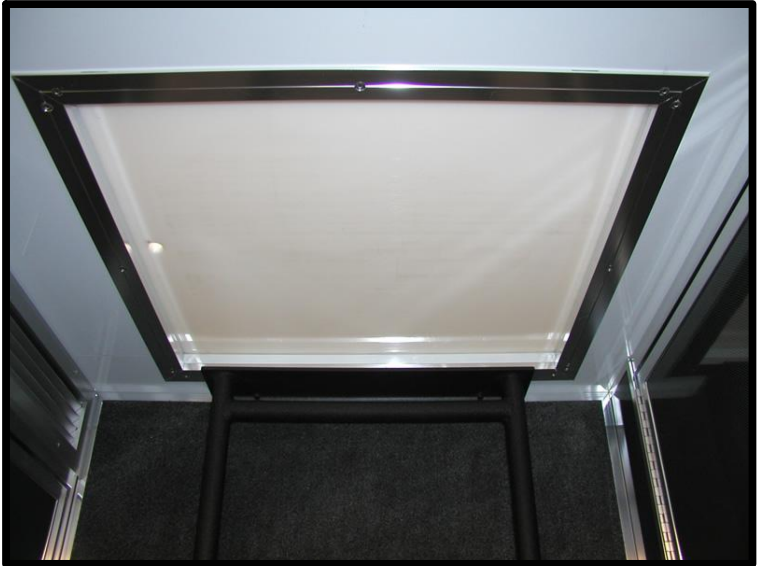
View of lower level ceiling at front wall – sliding access hatch to upper level
