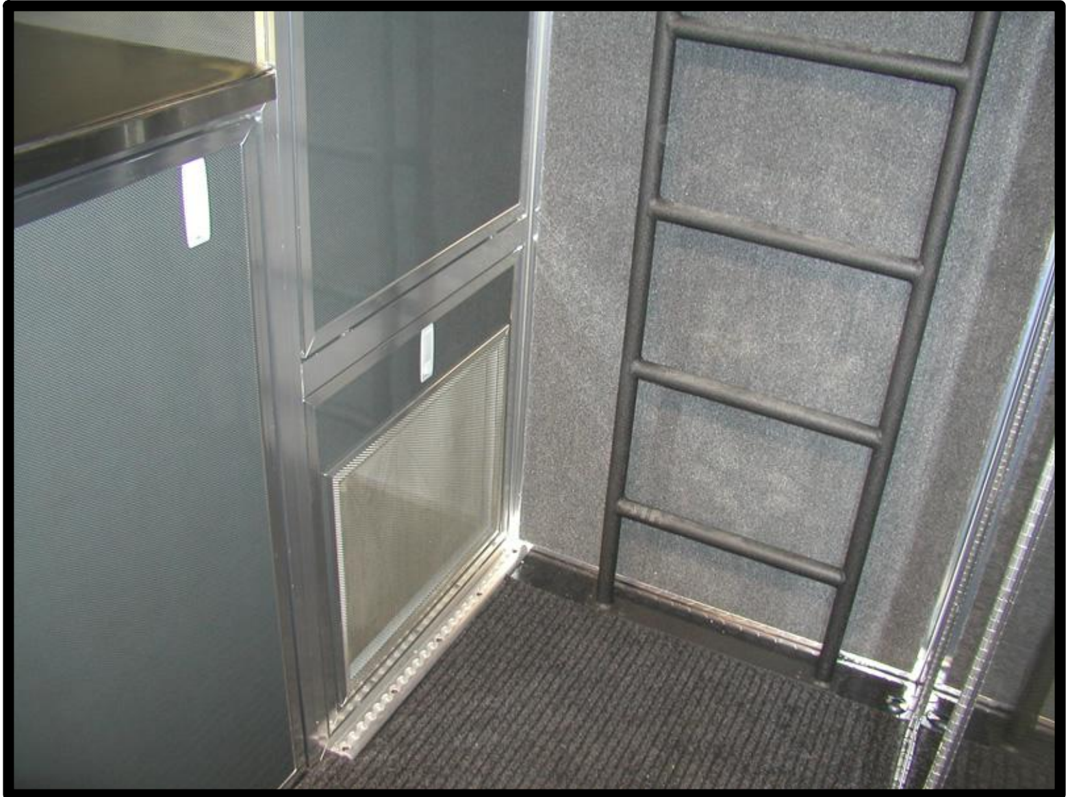
View of access ladder to attic level – A/C air handler cabinet is at left w/screen
