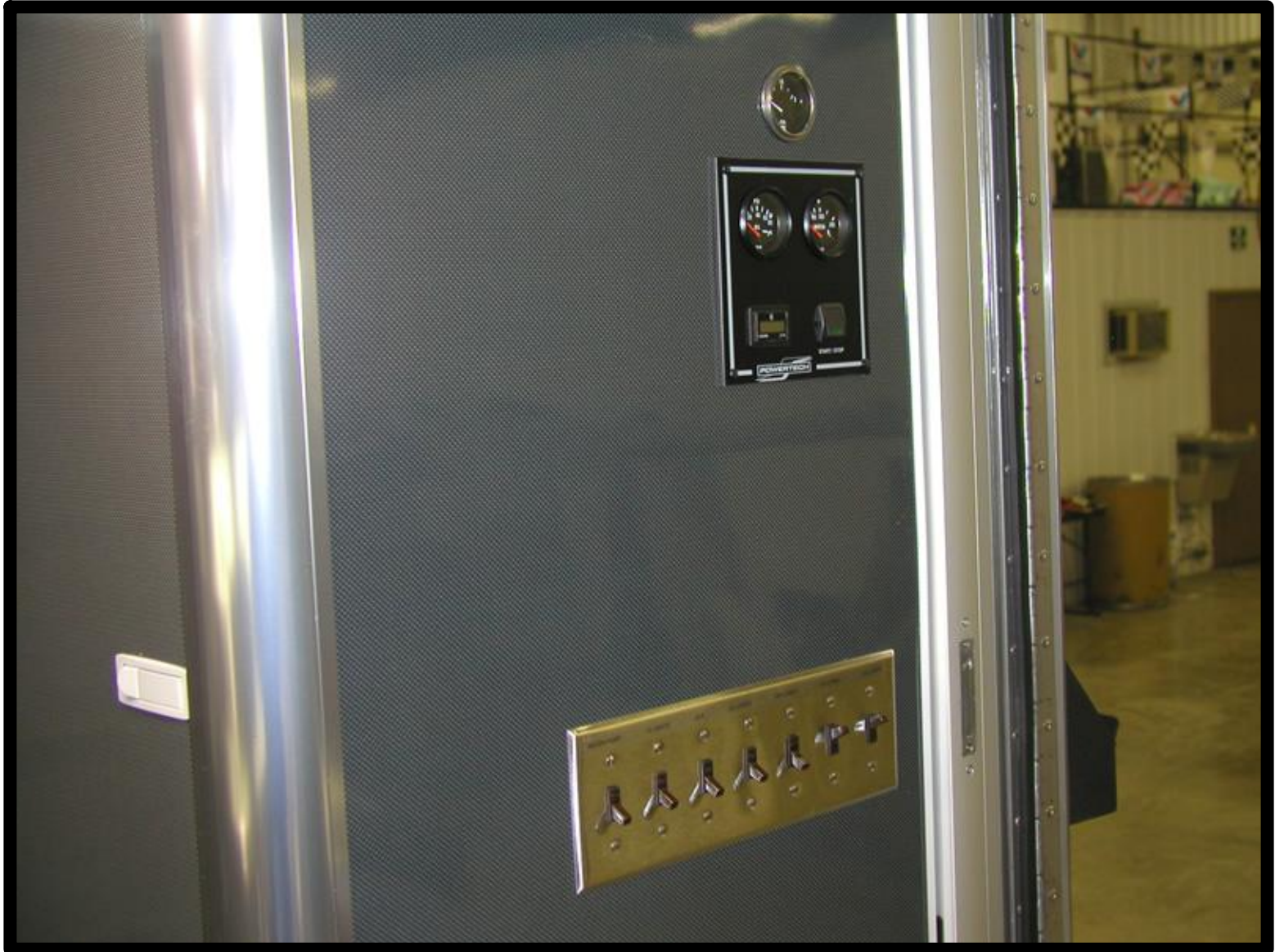
Lower work and storage area – switch and gen. gauge panels by main entry door
