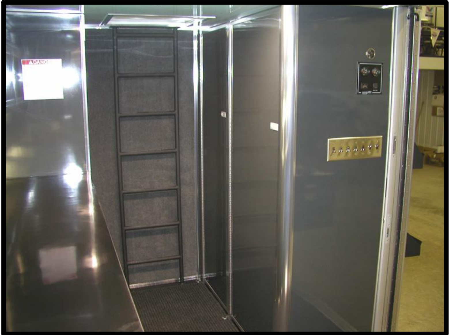
View of front portion of the work area inside trailer
